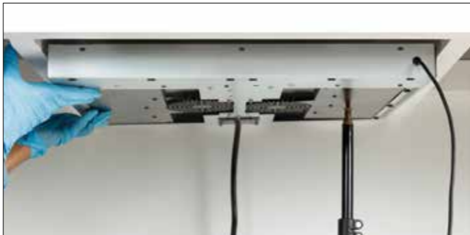
Using a prop, attach the system to the porcelain slab.
