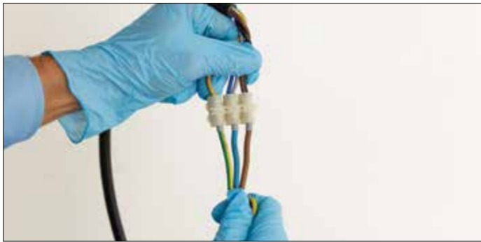
Connect the electrical cables and turn on the main switch. Finish assembling the furniture.
